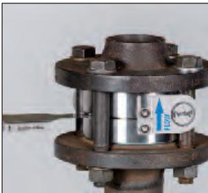
Combined with the REMBE IG-KUB holder the BT-IKB reverse acting bursting disc provides easy handling and an economical solution.
