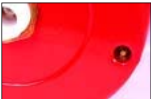
Bleed valve for rapid depressurisation and autodrain function check.
